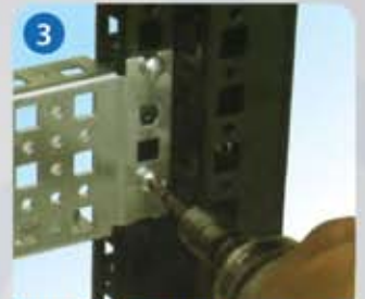
Installing Mounting Angle
